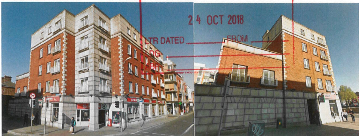
Figure 2.0 Image of the subject building at 'Chancery Hall' as viewed from Ellis Quay, Dublin 7.
