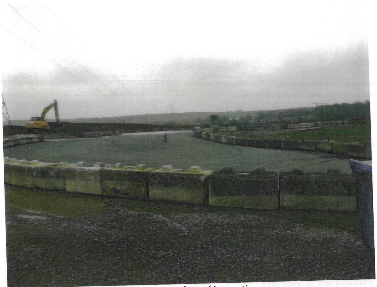
Track area. Excavator was functional on date of inspection
