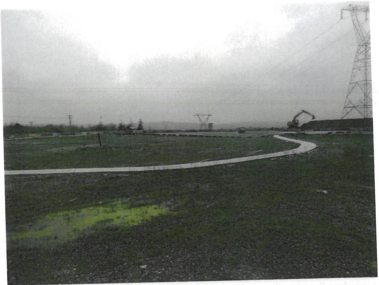
SE end of the site
