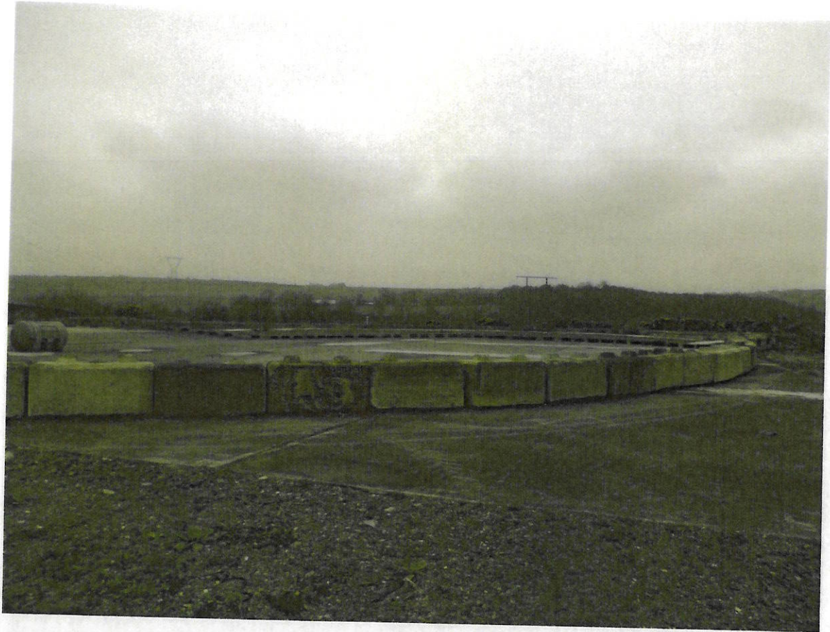
Southern end of track area
