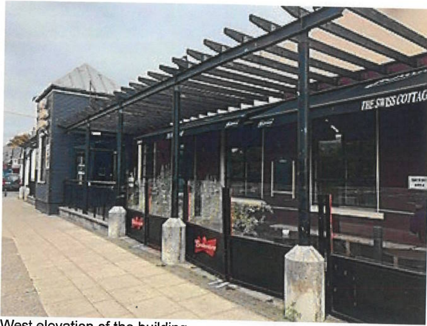
West elevation of the building
