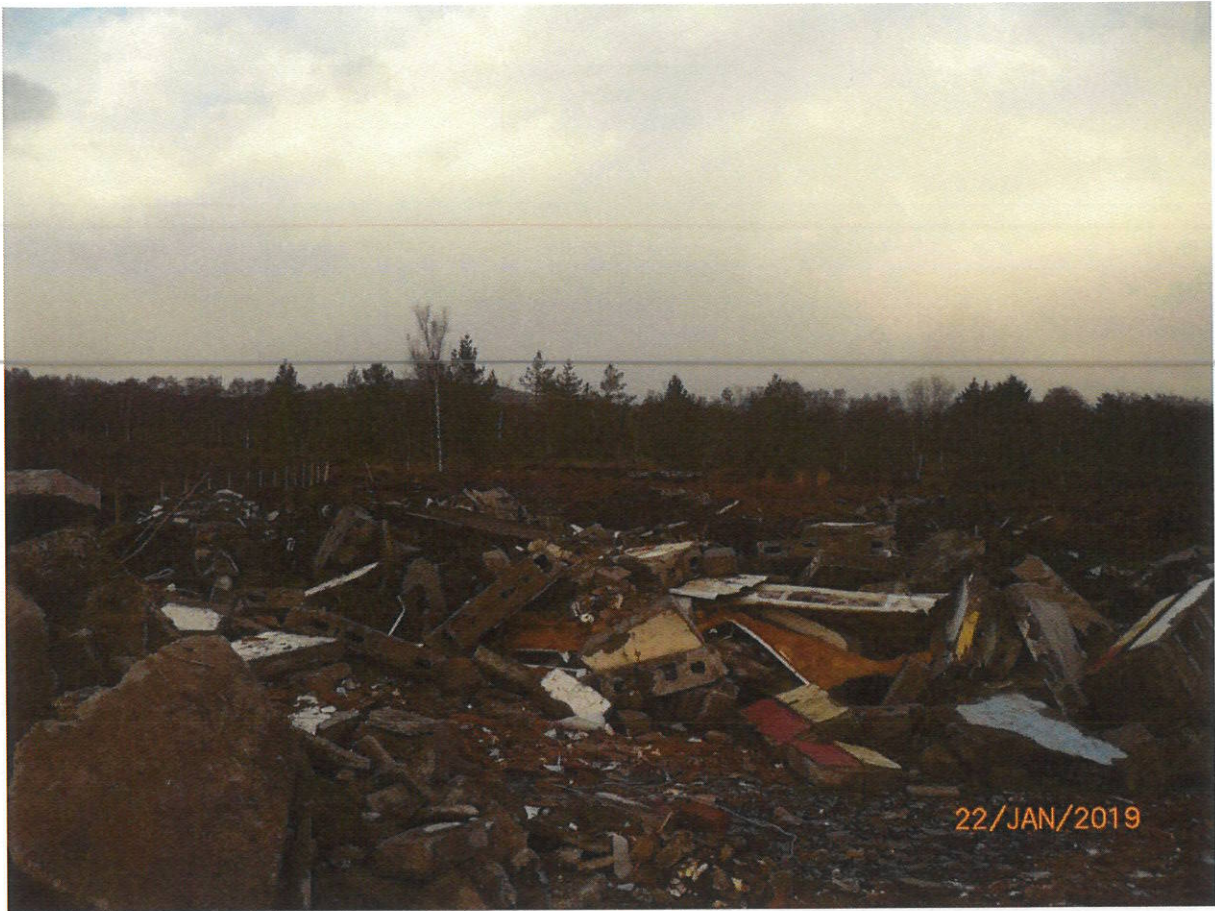
Photo No 13 – Unauthorised Clearance, Drainage, Importation of Construction & Demolition Waste and Filling in Bog Area
