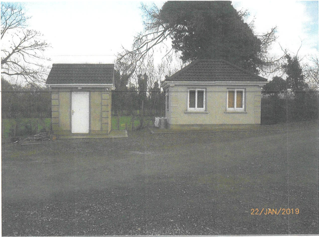
Photo No 1 Office and Toilet block at Entrance to Site
