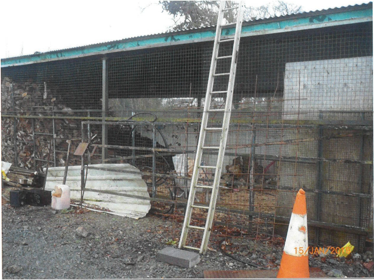
Photo No 7 - Timber storage Shed
