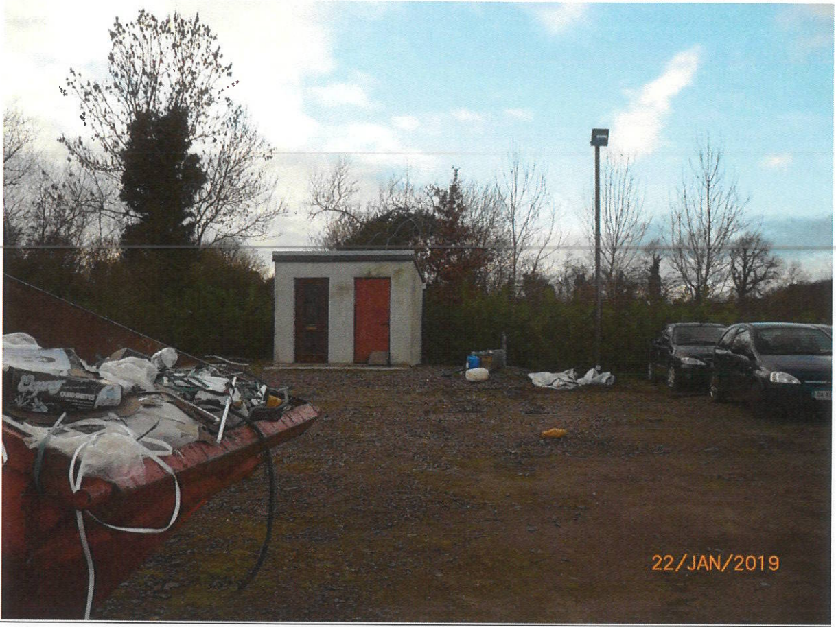
Photo No 3 Shed adjacent to Timber Cabin & Unauthorised Car Parking
