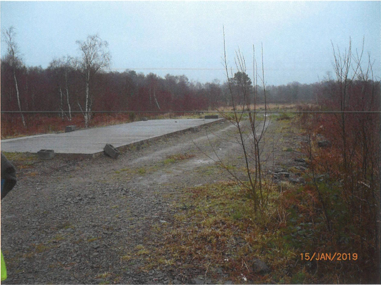
Photo No 14 - Unauthorised Concrete Slab in Bog Area
