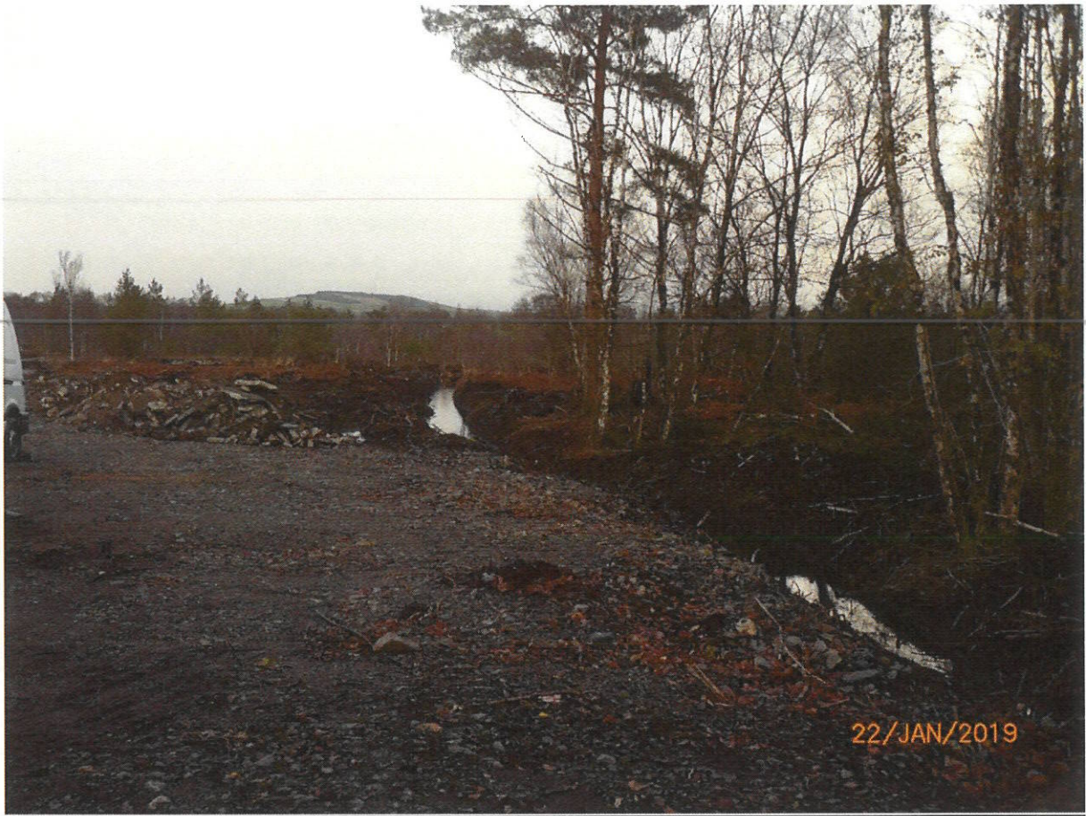
Photo No 11 - Clearance, Drainage & Filling of Bog
