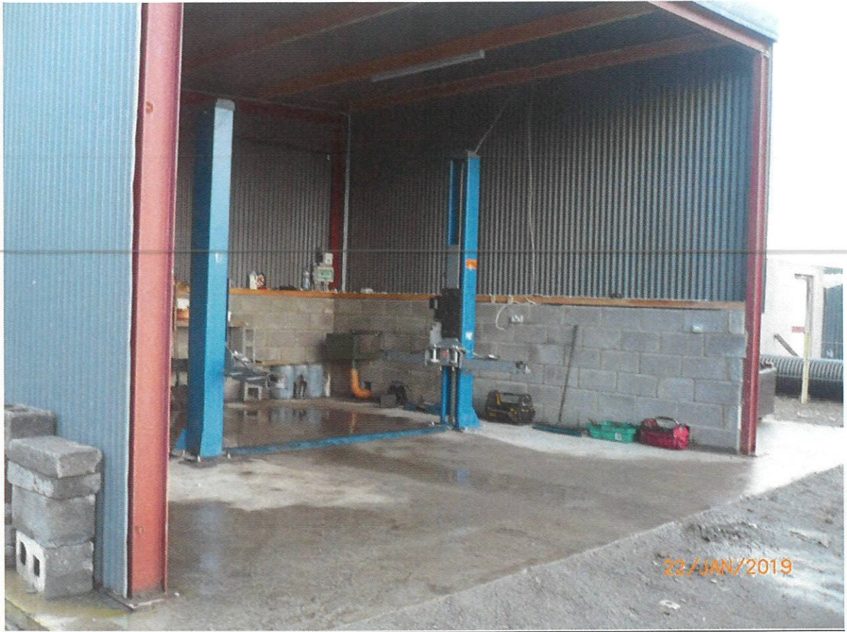
Photo No 8 - Shed containing Car lift & Toilet Block
