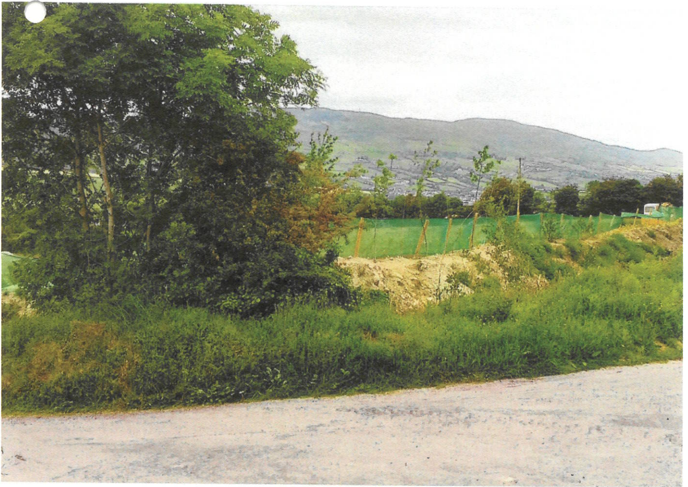
Image 2.4 Embankment, along southern boundary from road junction at S-W corner of landholding
