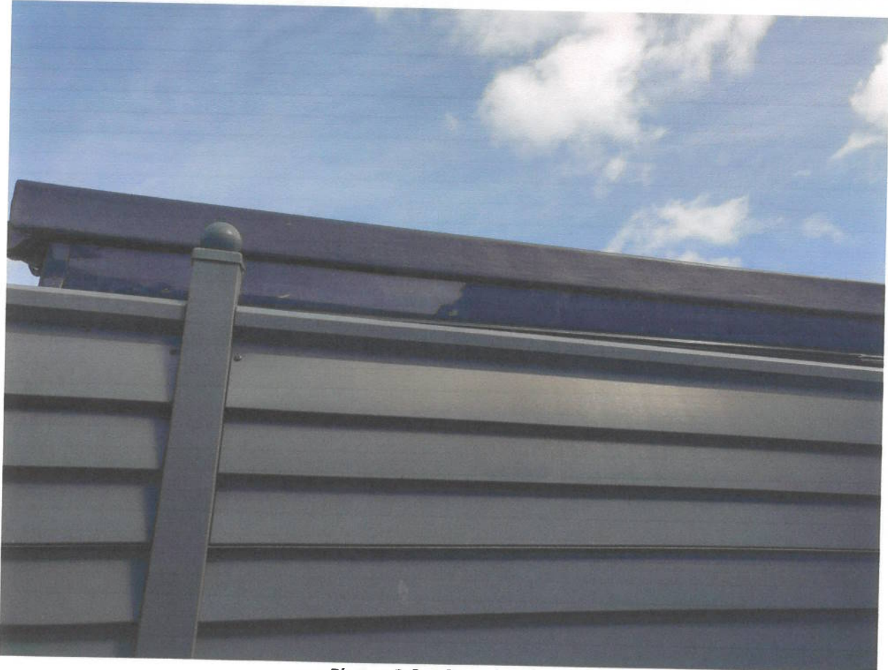
Photos 3 & 4 from South
