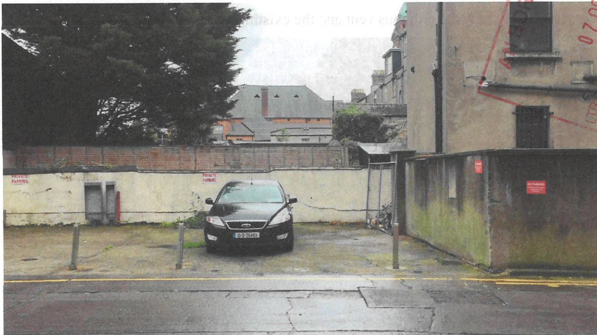
Image of New Ventilation Extractor Hood taken from Parker Hill
