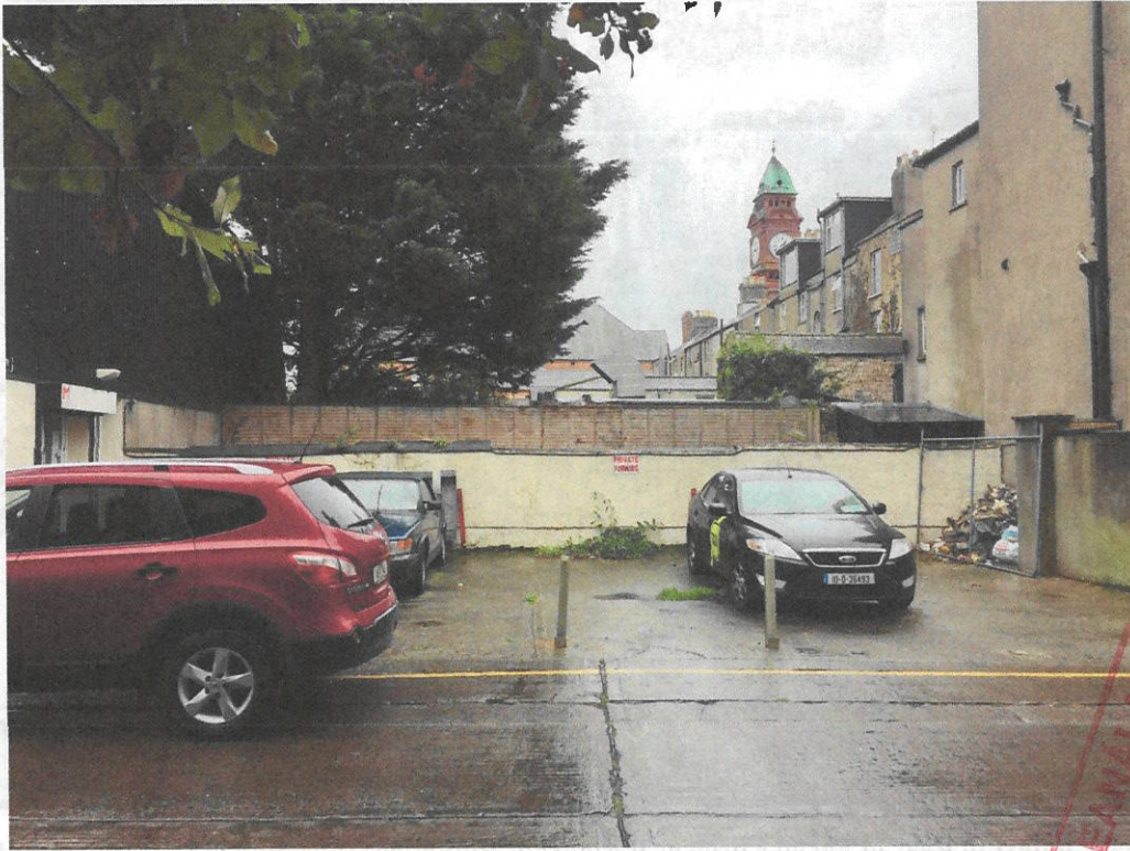
Photograph of New Ventilation Extractor Hood taken from Parker Hill
