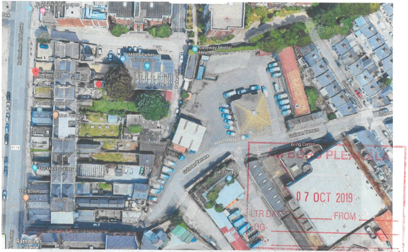
Commercial Context to Rear of Farmer browns Restaurant Rathmines (Location of Extractor Hood marked with Red Dot)
