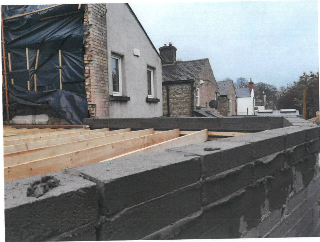
Photograph 5 – taken 4 April 2019, showing the start of joisting out the single-storey roof. These subsequently removed prior to building double-storey height.
