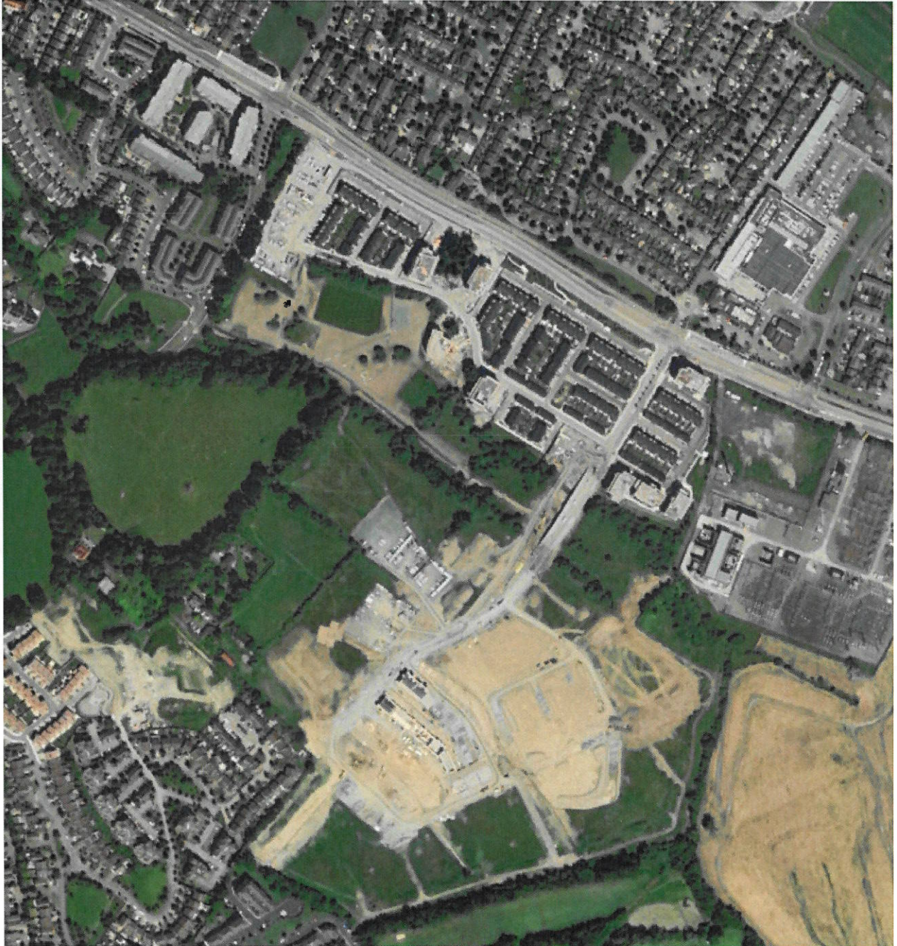
Figure 3 - Aerial Photography March 2019, showing progress on eastern section of Loop Road
