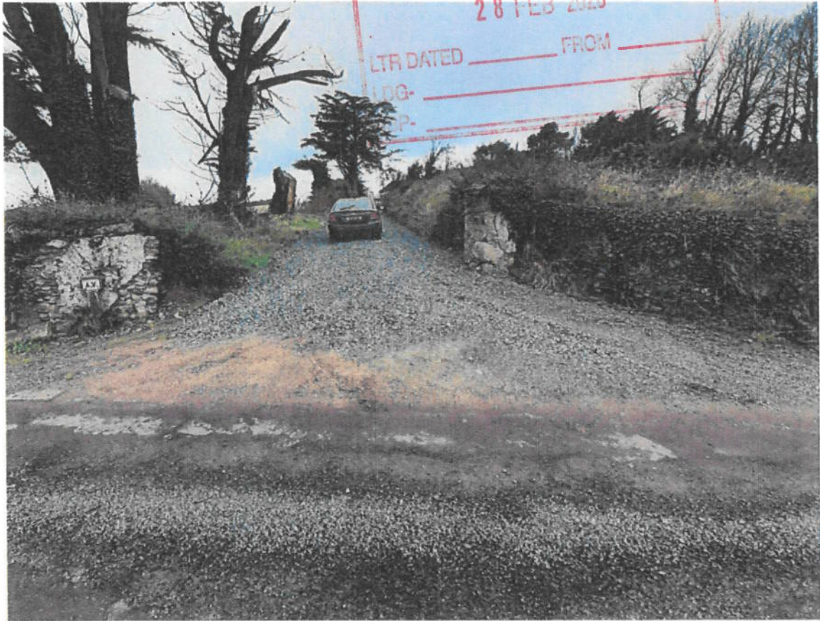
Fig: Entranceway and re-surfacing work, 24/01/2020. ✓
