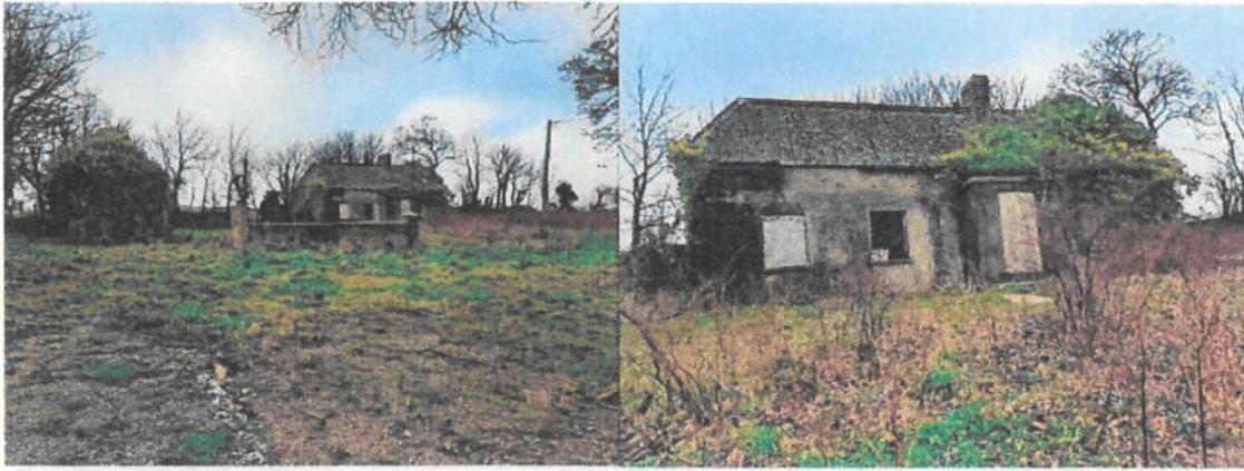
Fig: Derelict Dwellinghouse to rear of laneway, c.250m from access to public road. Part of infilled marlhole in photograph to LHS
