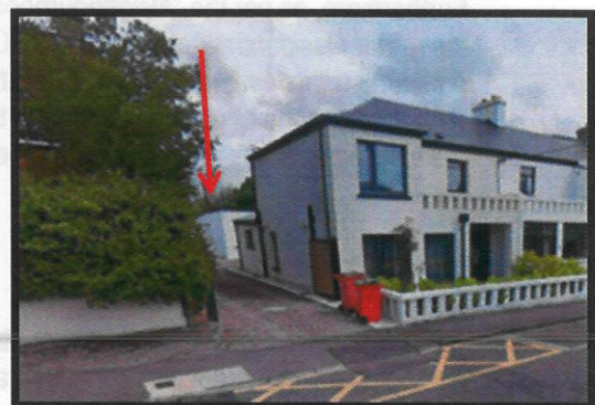
Figure 4: Photo of No. 31 from Shantalla road
