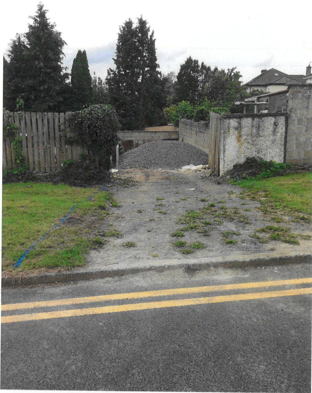
25 th June 13:56. Ground marked out by Building Contractor for 14ft wide vehicular entrance.
