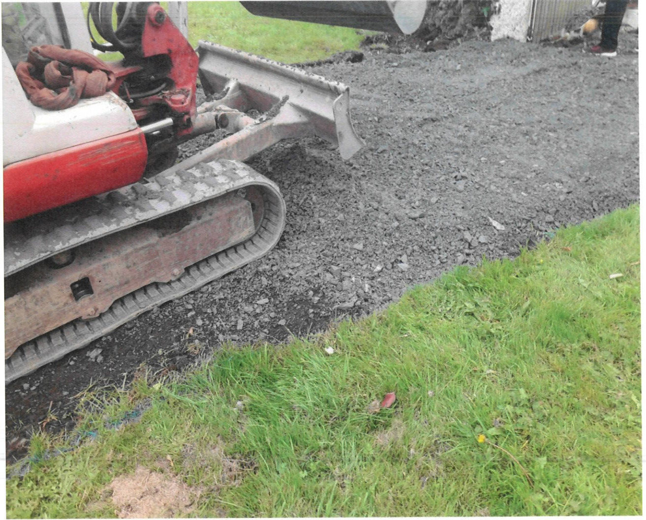
30 June 2020 19:14. Excavator spreading and compacting gravel.
