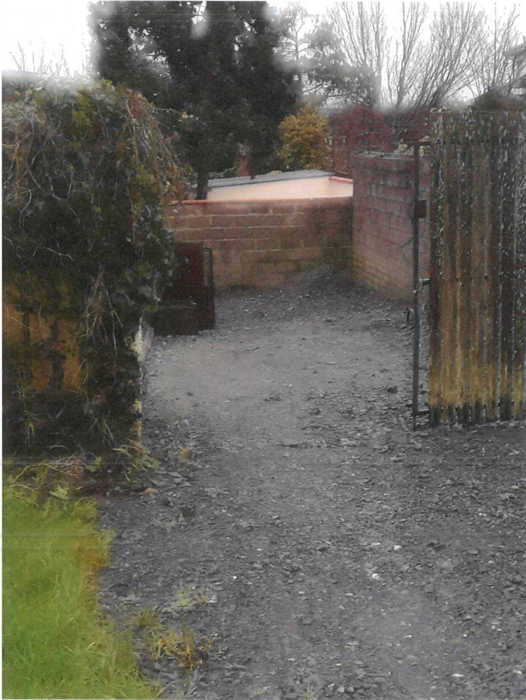
23 rd December 2020. Resulting outcome of gravel loads delivered by this date.
