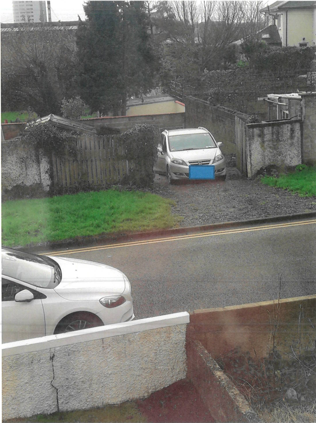
1 st December 2020 11:53. Strandville Gardens neighbour delivering gravel to site using unauthorised driveway.
