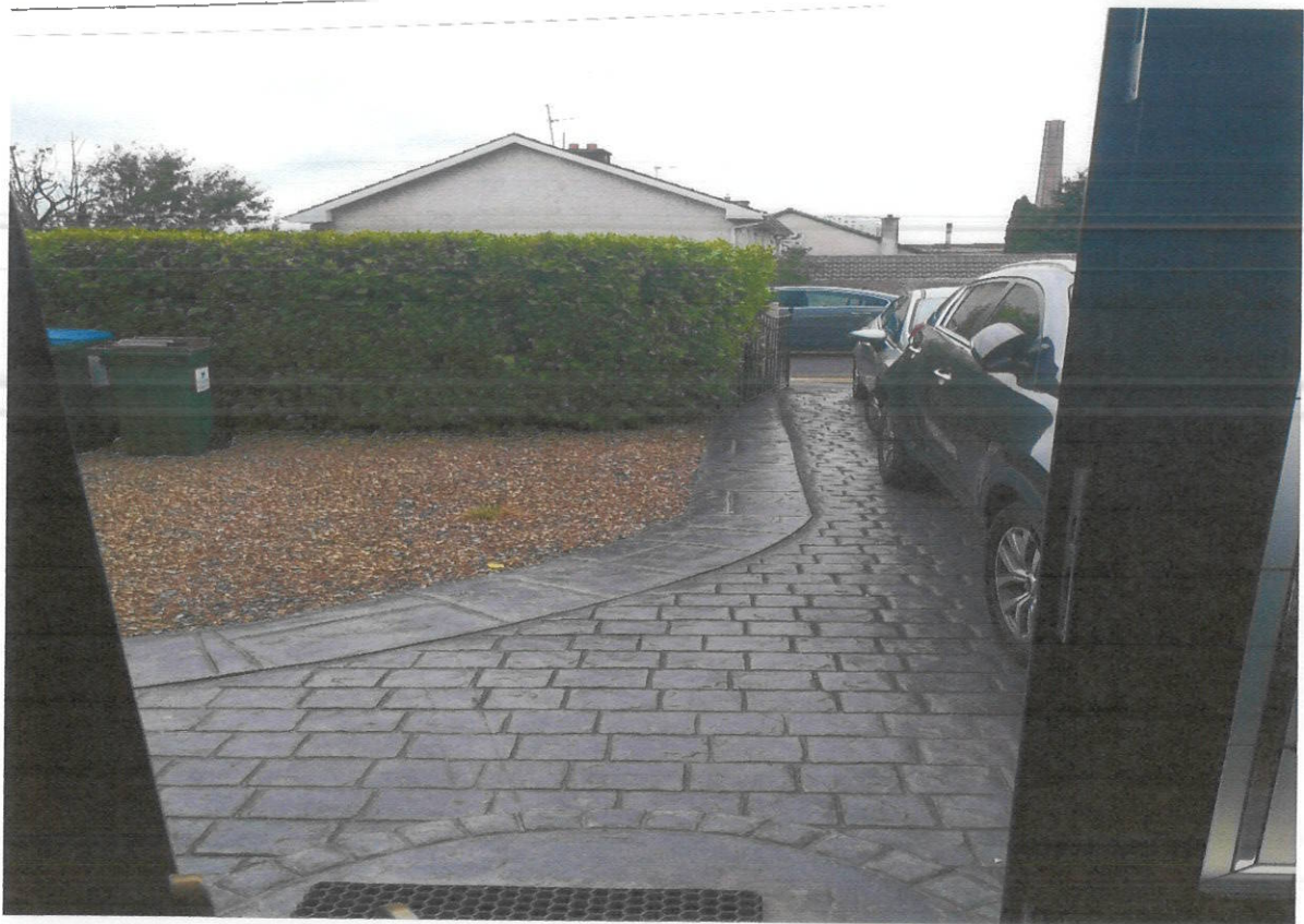
Exit from homes blocked.
