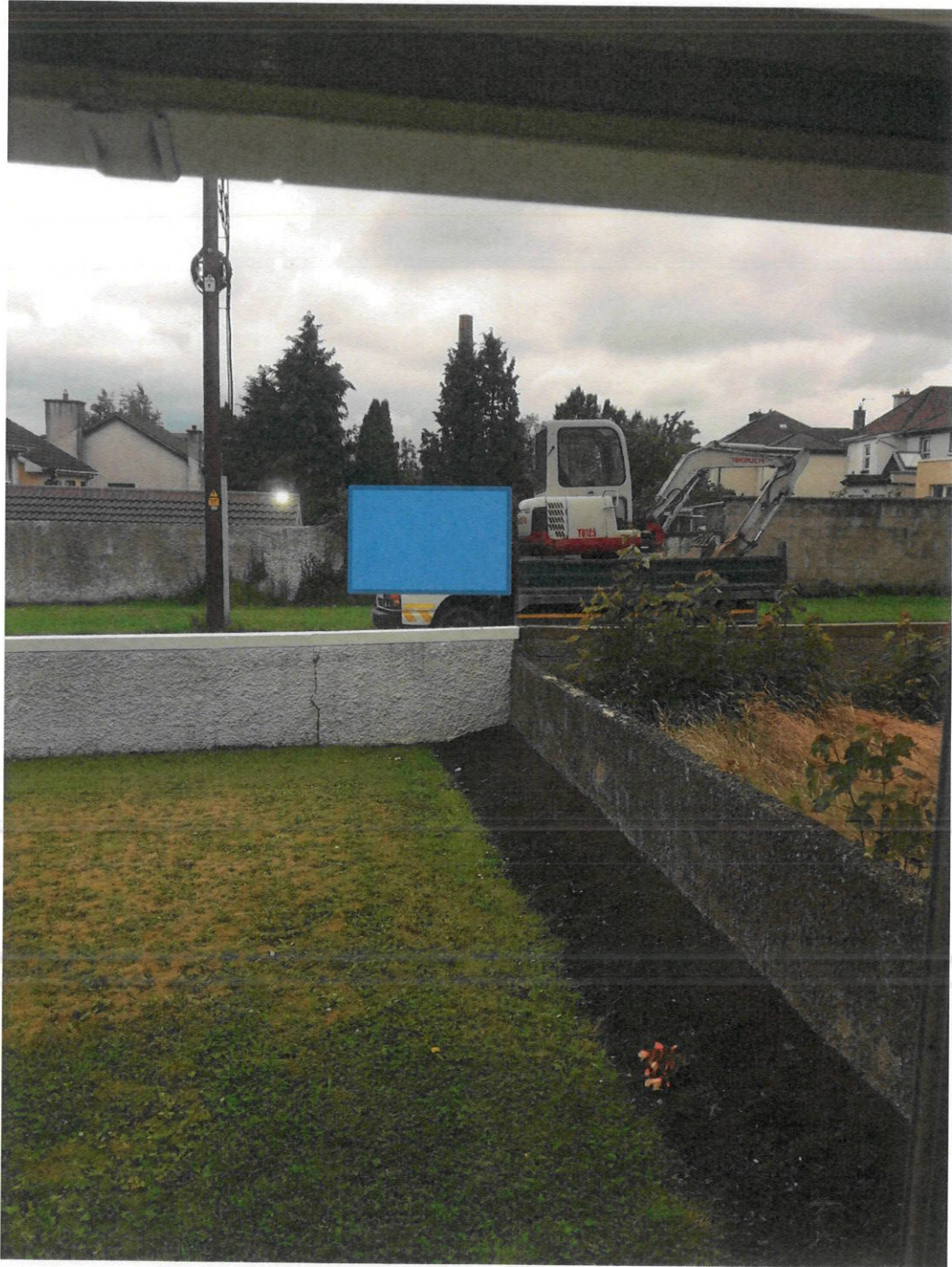
30 June 2020 18:18. Excavator arrives.
