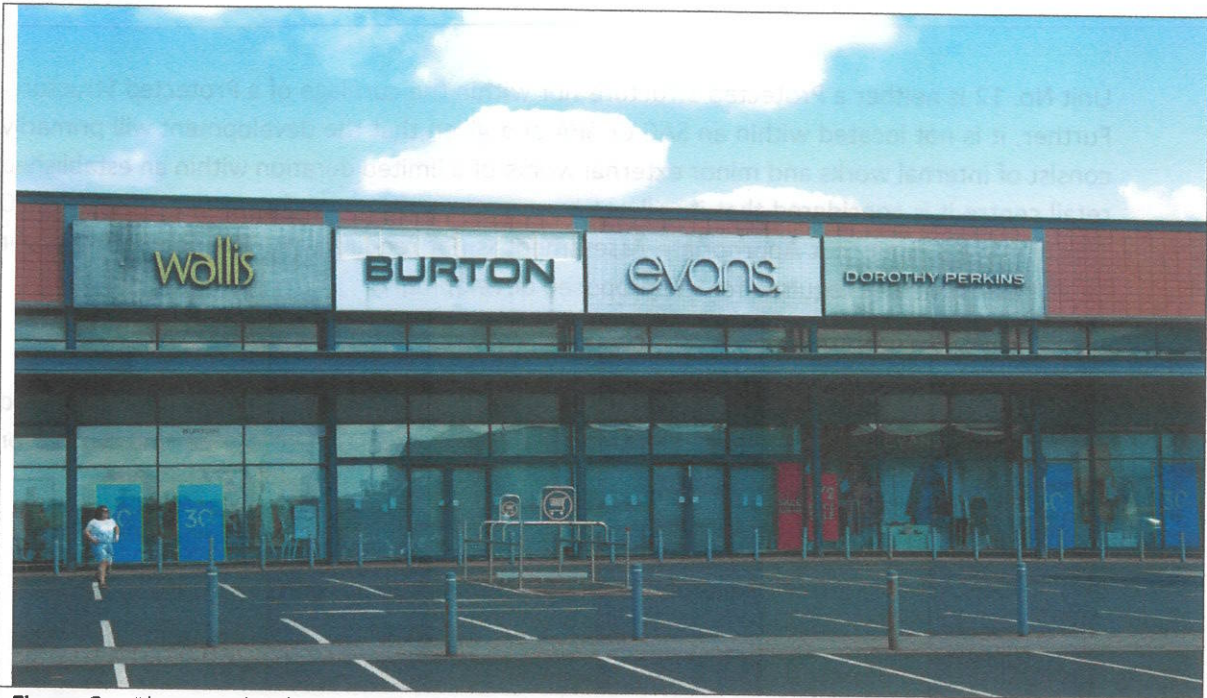
Figure 2: Photograph of the entrances to Unit No. 12 located on the southern elevation. Under the scenario/proposal 1, additional entrances/doors would be installed in the glass façade at the location shown on Drawing no. P-1202 (please see the drawing relating to scenario 1 only) and also at the rear elevation. The size of the entrances and the materials to be used would mirror those of the existing entrances. Source: SheehanPlanning
