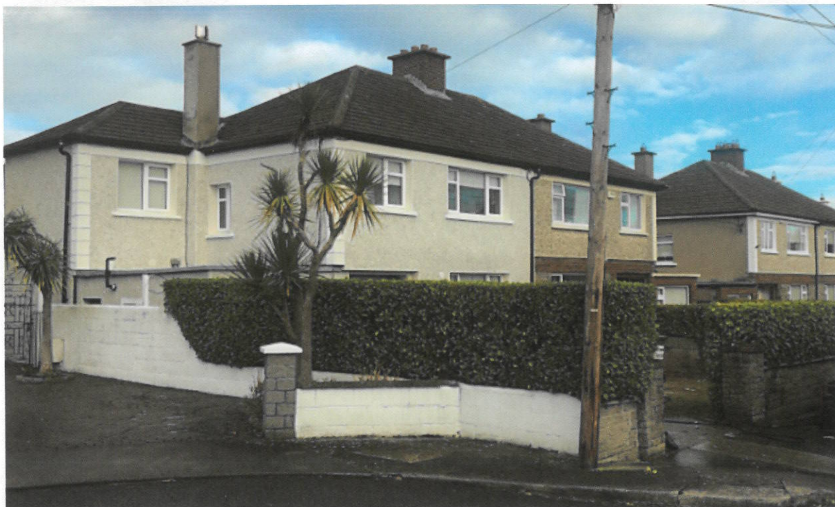
Photograph 8: The alterations to the referral property are immediately apparent from the street (compare with its previous appearance in image no. 4 above).
