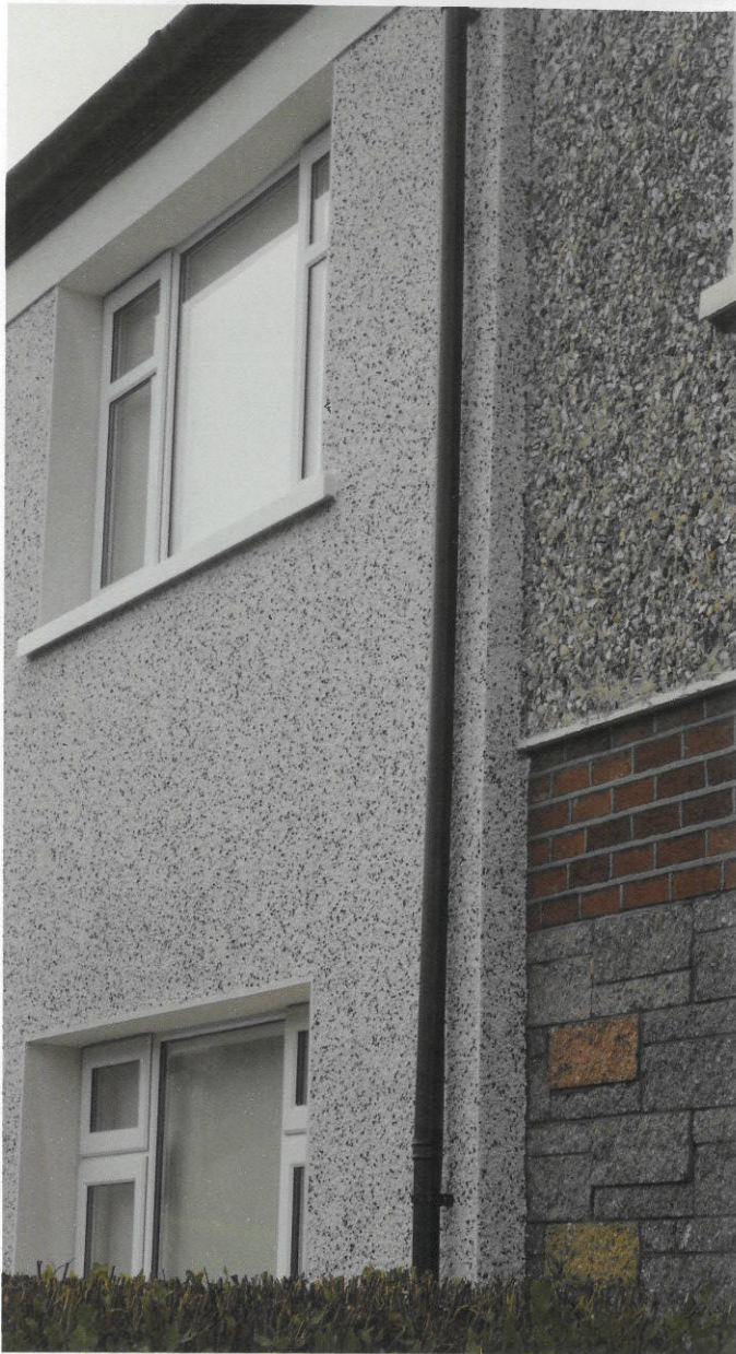
Photograph 7: The front projection to the façade of the referral house.
