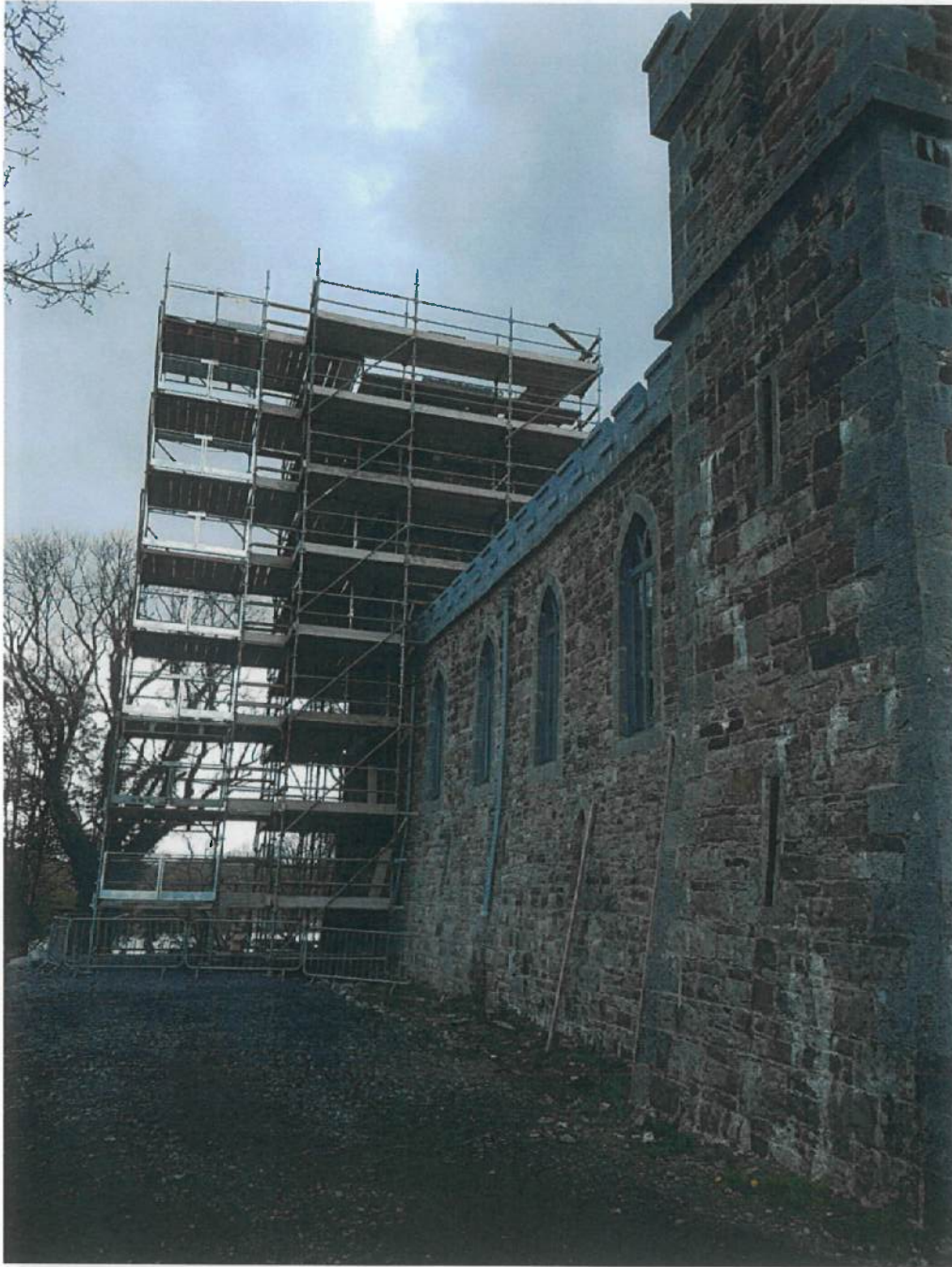
Photograph 1 – taken at side of building – Note scaffolding around ‘high tower’.
