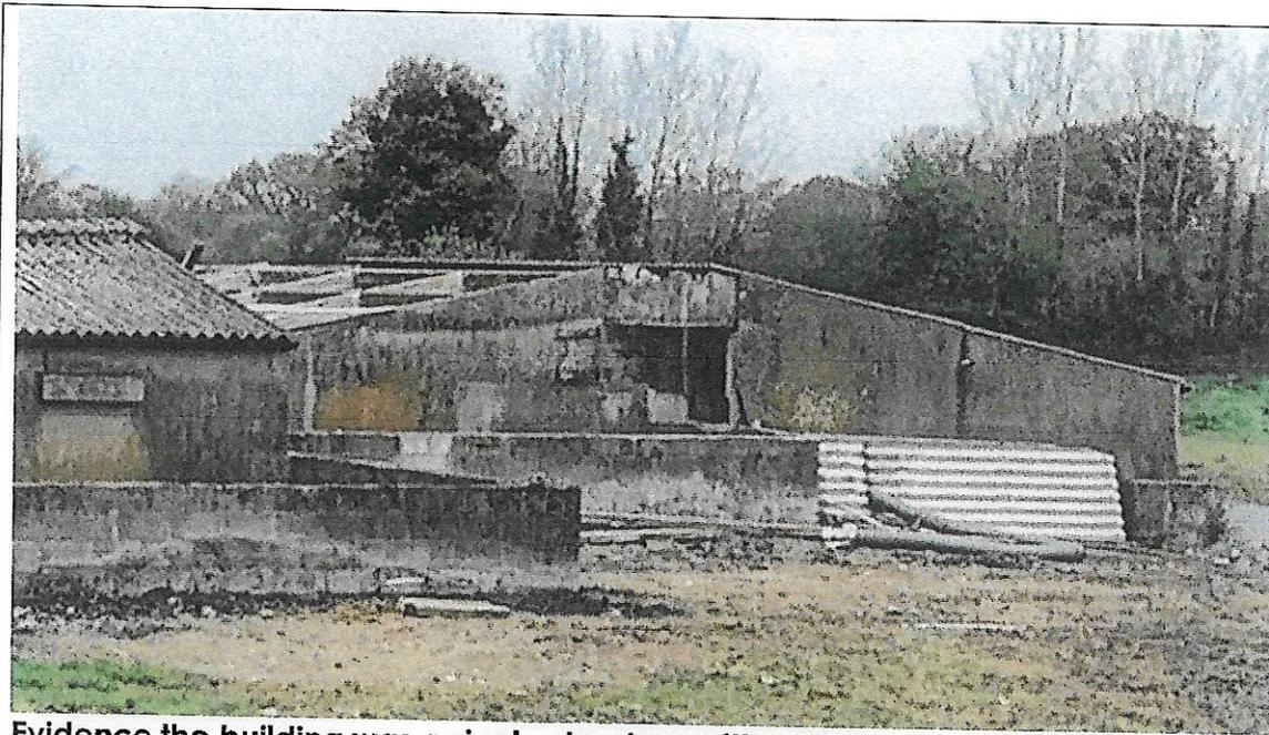
**Evidence the building was a single structure with bridging over the gable door.**
