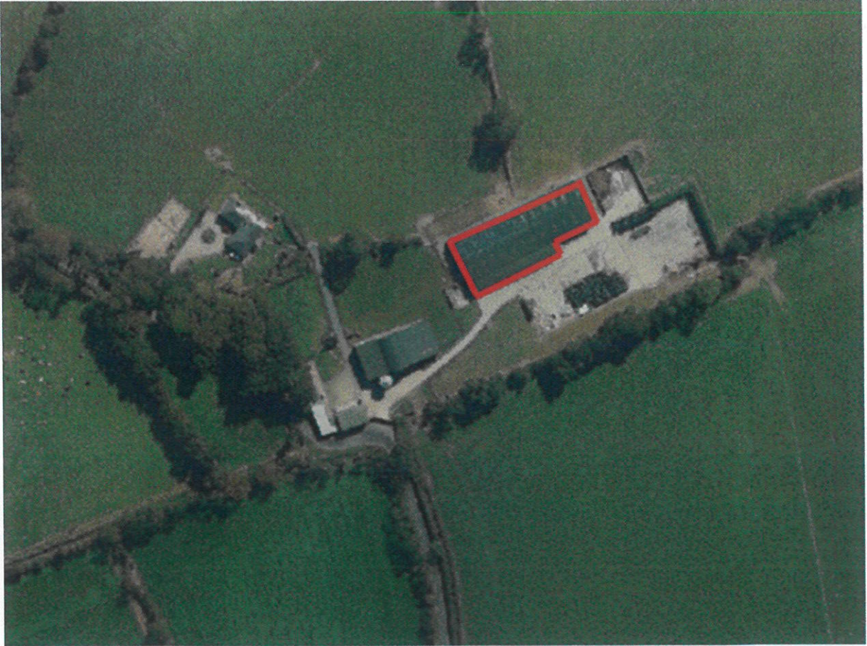
Shed for which this declaration is being made is being made in red below
