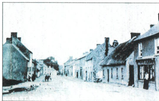
View of Mary Street (formerly Queen Street) c. 1900. At least two buildings in the photograph have thatched roofs. (Source: O'Doherty)
