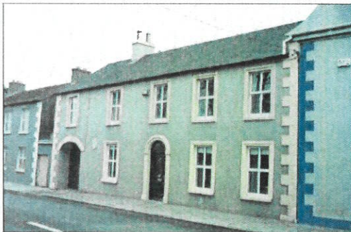
Building displaying moulded render window and door surrounds and channelled quoins, Castle Street
