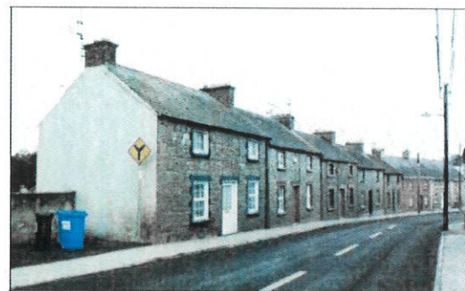
Stepped roofline following natural slope along Carrigan Street.
