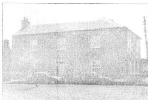
Photo 9 The Former Courthouse on The Green
