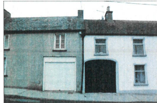
The alteration of openings and the insertion of modern doors results in slow erosion of the characteristic features of an area.
