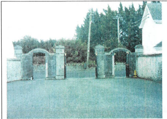
Gates to Brittas Demesne
