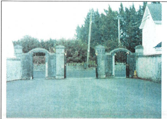
Gates to Brittas Demesne
