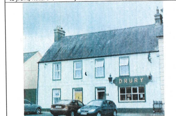
Traditional shophouse with stained glass lantern, with living quarters to the side and above
