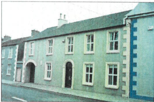
Building displaying moulded render window and door surrounds and channelled quoins, Castle Street
