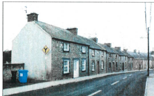
Stepped roofing following natural slope along Carrigan Street
