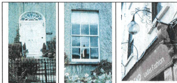
Surviving historic building fabric: painted timber door with decorative fanlight; timber sliding sash window with crown glass; decorative painted console
