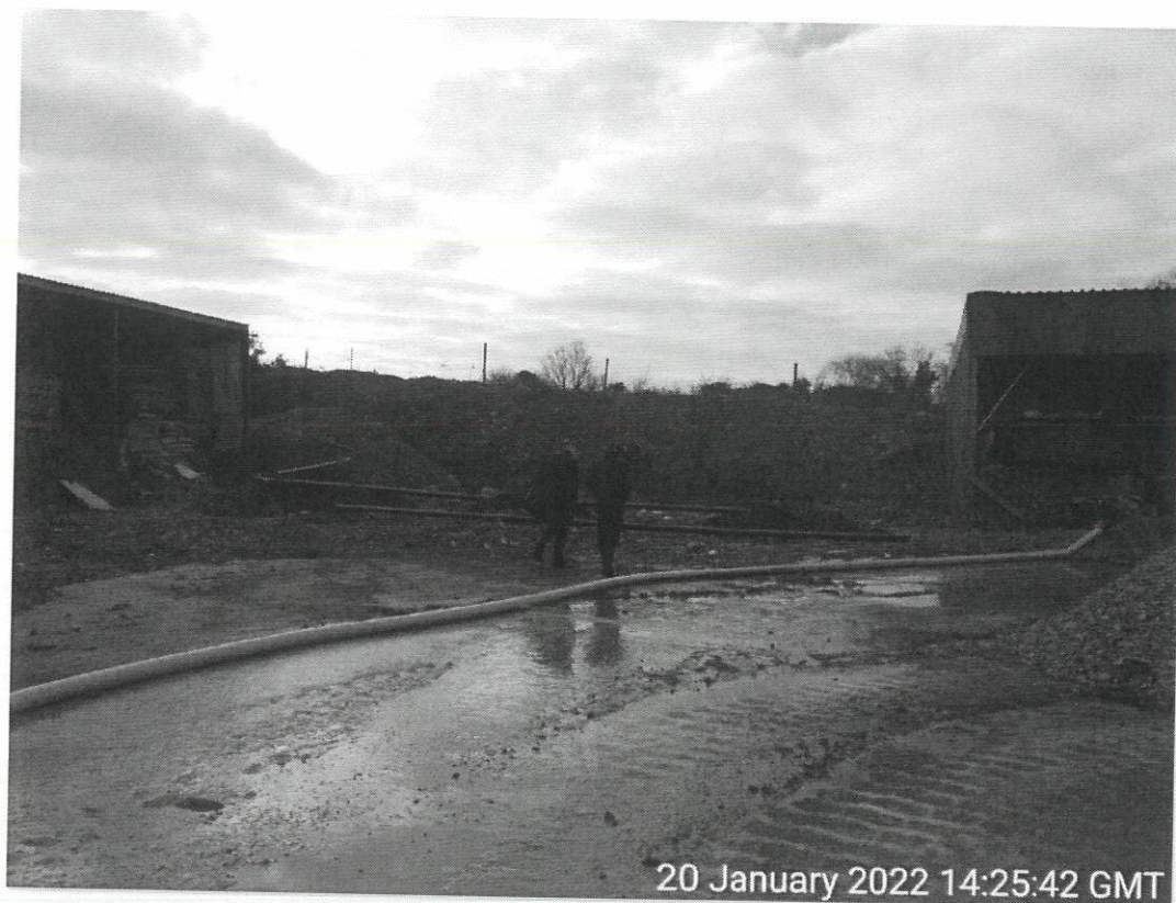
Photo 9-11: Yellow pipe running from lagoon system out of site to road. Black piping in situ adjacent to soakaway, including additional pipe to facilitate additional water discharge.
