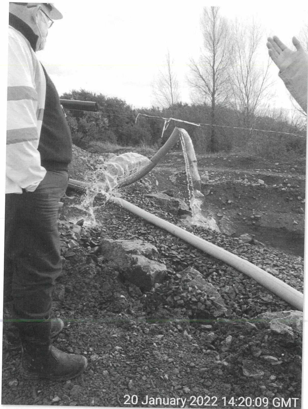
Photo 4: Water discharging into lagoon system and directly out of site via yellow pipe.
