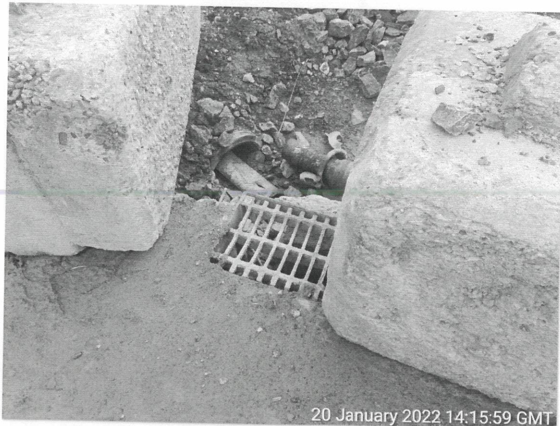
Photo 3: Alleged old pipe and drain gully in situ.
