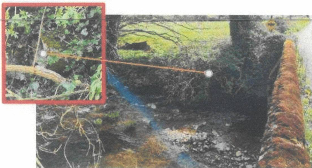
Plate 5 Discharge pipe into Nenagh river from gully at site entrance
