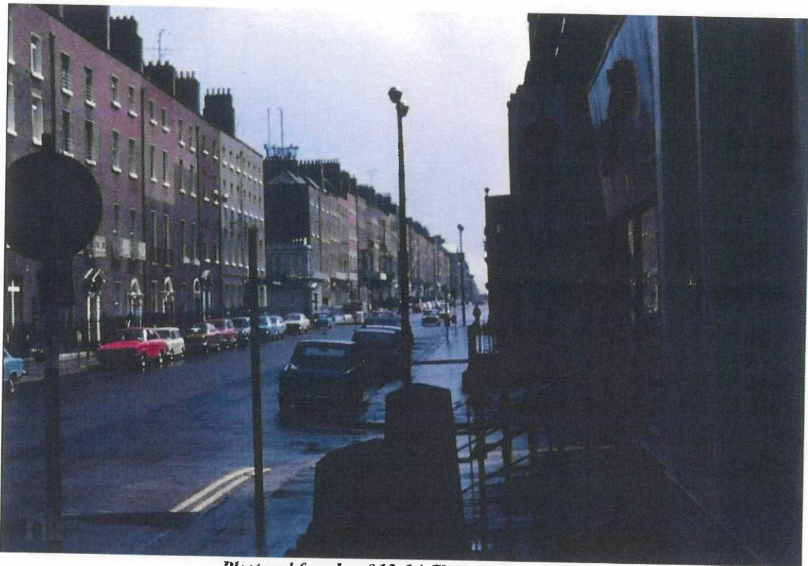
Plastered facade of 13-14 Clare Street - 1972
