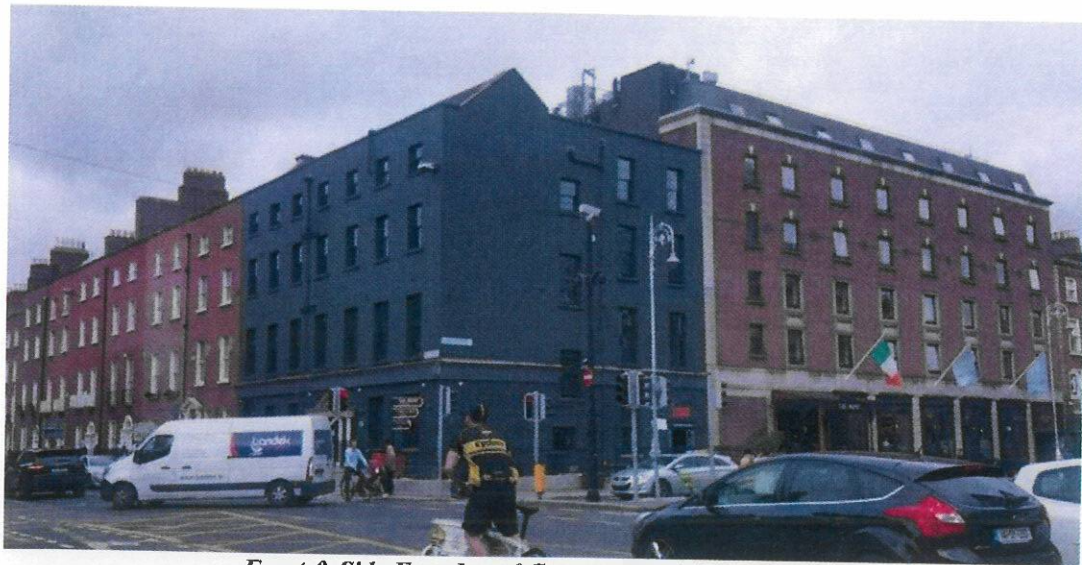
Front & Side Facades of Current Hotel Paint Colour
