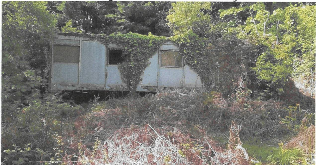
Plate 1 – Foreground Area of Levelled Access 'Overgrown'
