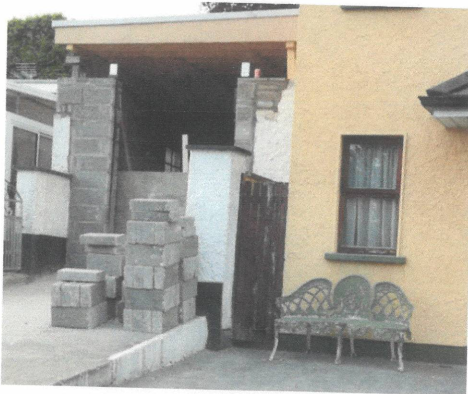
Plate 3 Works being carried out illustrating change in roof profile
