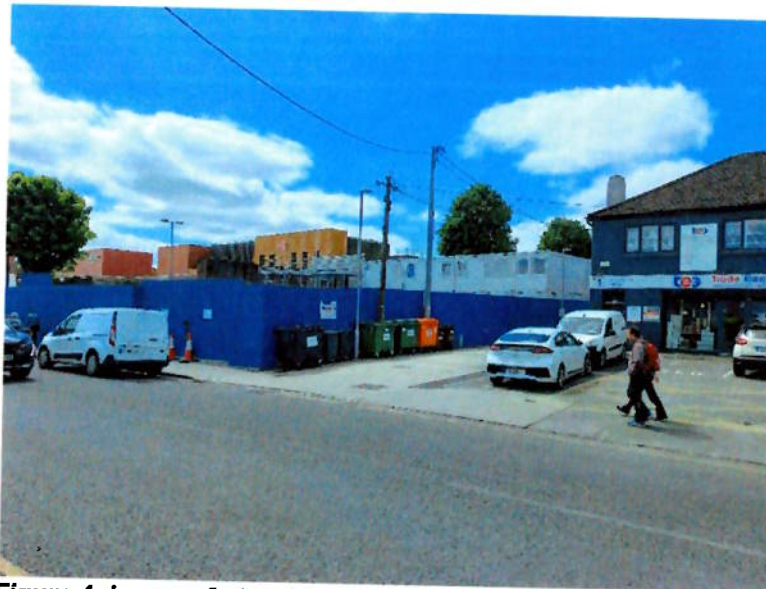
Figure 4: Image of structures on site.
