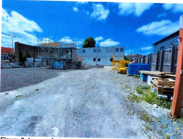
Figure 3: Image of structures on site.
