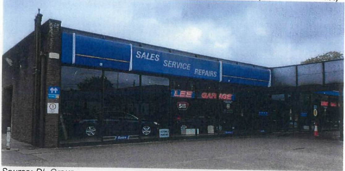
Figure 2.2: Photo of Lee Auto Centre car sale showrooms (east of forecourt)
