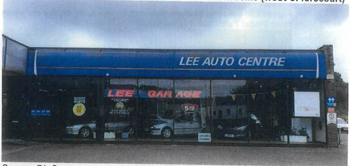
Figure 2.3: Photo of Lee Auto Centre car sale showrooms (west of forecourt)
