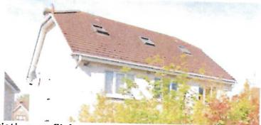
View of 3no. Existing rooflights to rear of No. 16 showing openable sections
