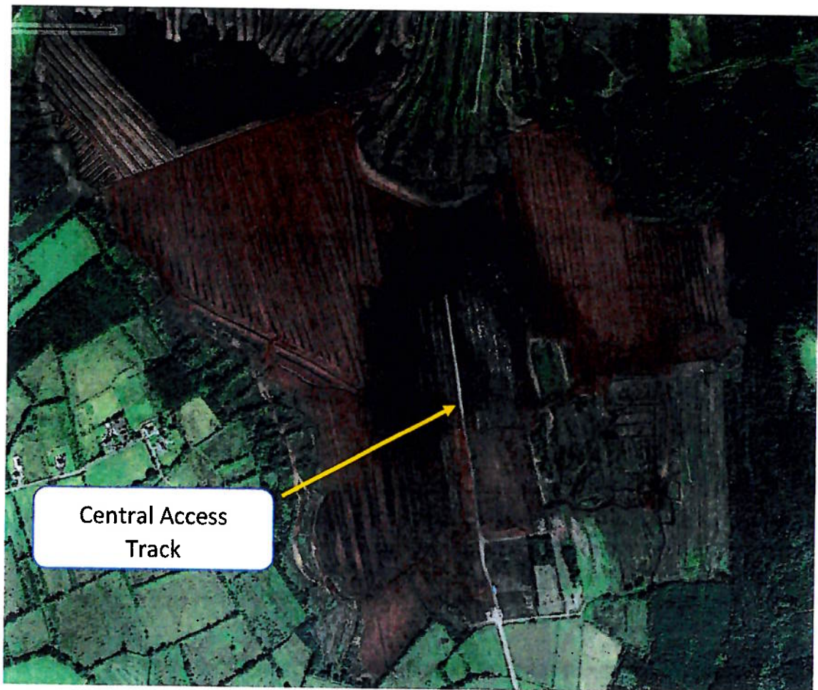
Figure 1: Aerial image of Derrymore Bog, generated from drone-based survey, reported by Brandon O'Brien Consulting Engineers (Church Street, Roscommon F43 P661), April 2023. The grey colouration in the centre of the bog reflects the exposure of the peat substrate. Once the substrate is encountered in drain beds in an area, peat harvesting ceases.
