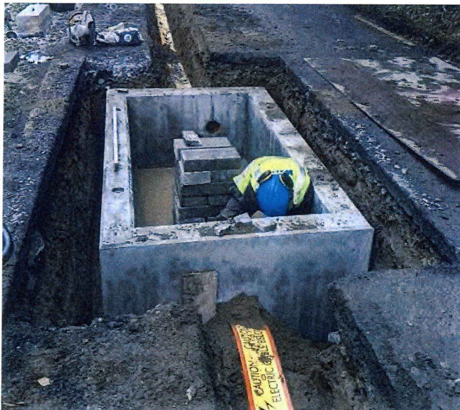
Figure 08 - Typical example of a 20kv Joint Bay in a public road.
