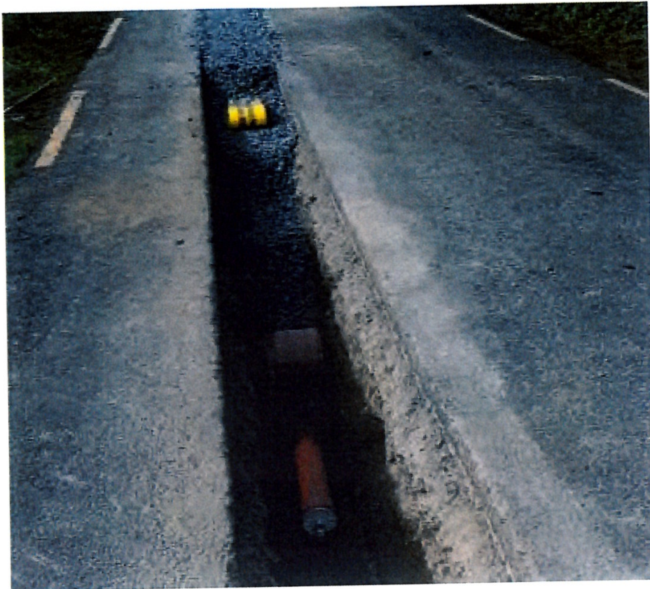
Figure 04 - Typical 20Kv Trench Profile &amp; Back fill
