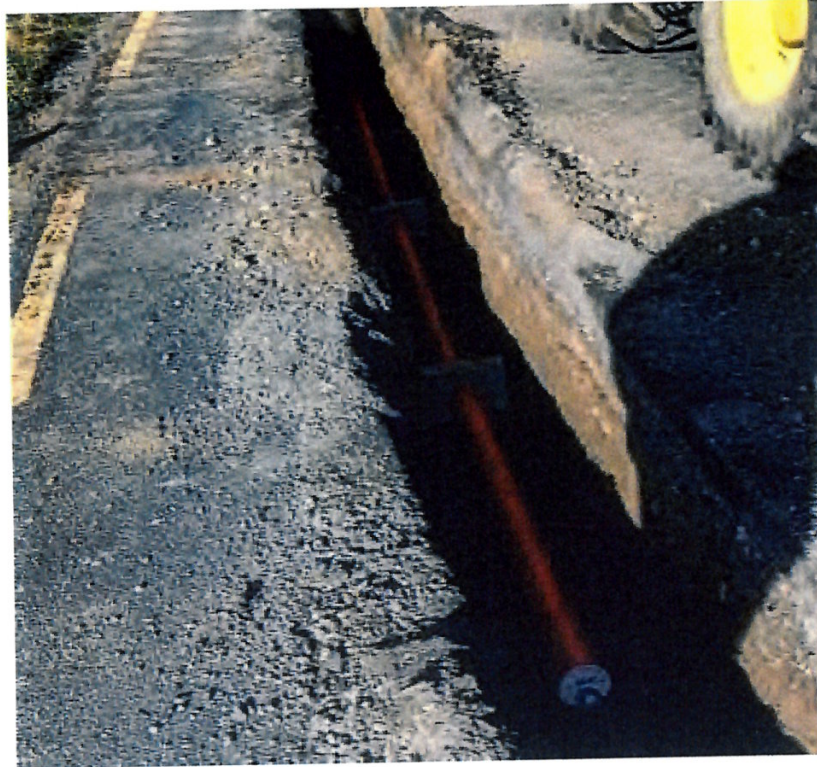
Figure 03 - Photographic Example 20Kv Duct Laying in a public road, ready for back filling
