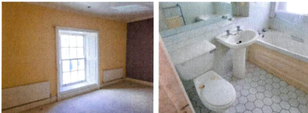
Figure 6.0 A first-floor bedroom and bathroom in Hayden's Hotel, as included in the photographic survey carried out on 1 st April 2025.
