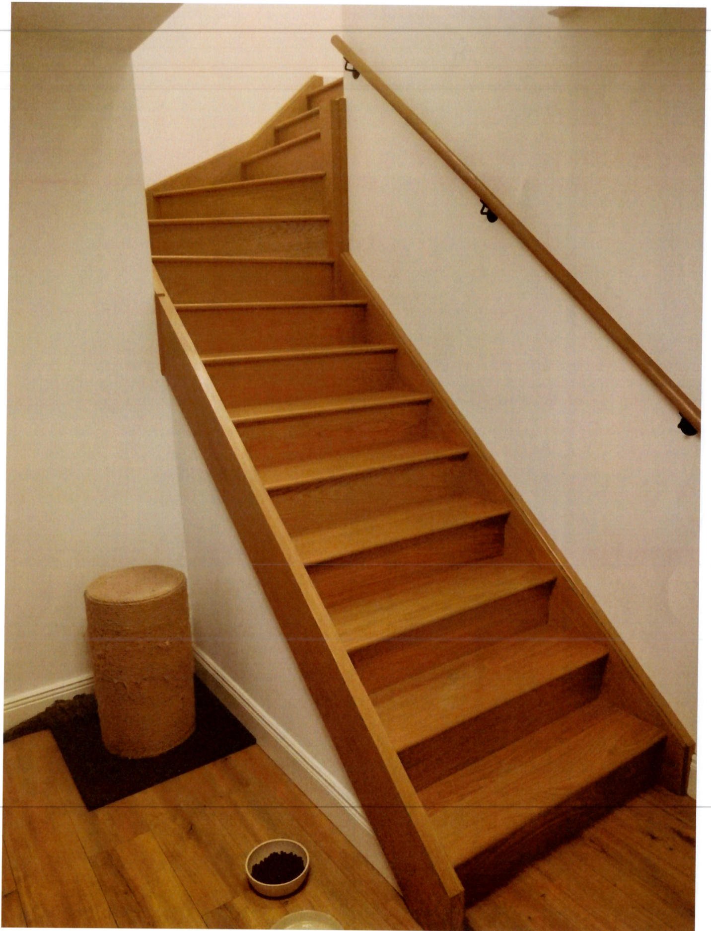
STAIRS leading to sitting Room Bathroom was Removed to install these STAIRS
