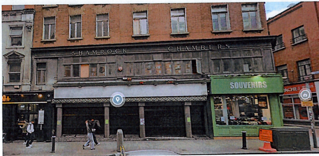
Figure 4.3: Previous Shopfront before Improvement Work Carried Out
