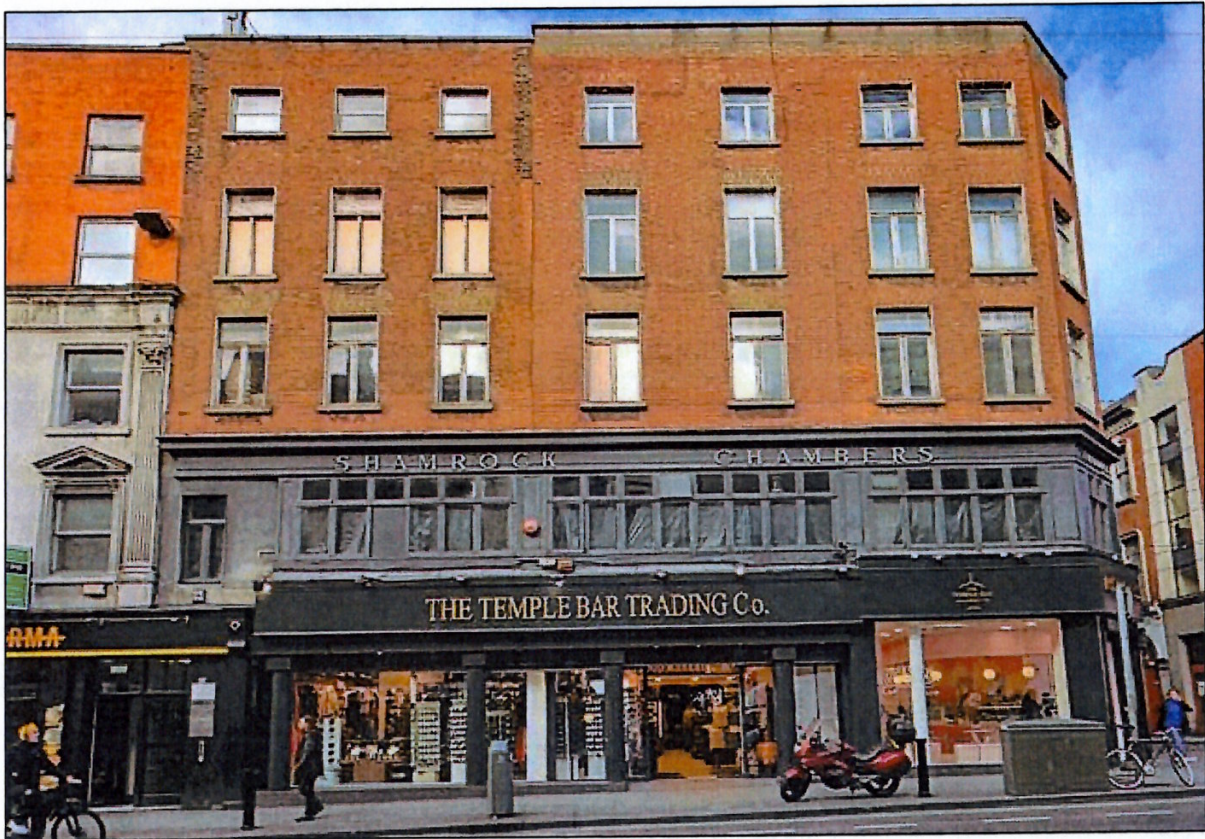
Figure 4.3: Shopfront after Maintenance and Improvement Works Carried out
